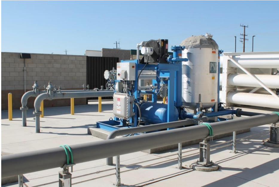
Photos: – CNG Dryer System (top) & Completed CNG Station (bottom)
