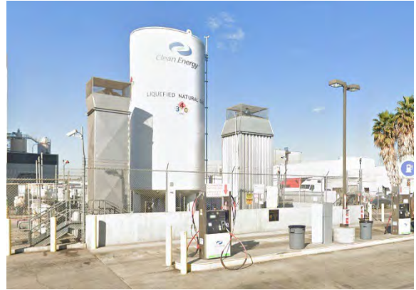
City of Commerce L/CNG fueling station on Sheila Street
